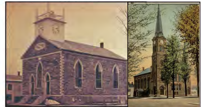
Images (L): First church building of stone masonry construction with both Federal and Gothic Revival style detailing. Church faced Lincklaen Street. LSHS
