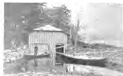
Figure 8. Oaks Boathouse during construction. Note stone dam on the right (photo from Upland 96).
